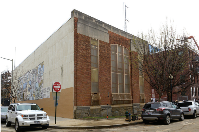
Current Champlain Substation
