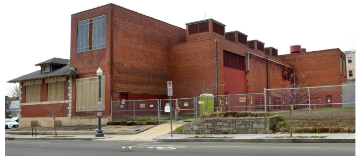
Current Harvard Substation
